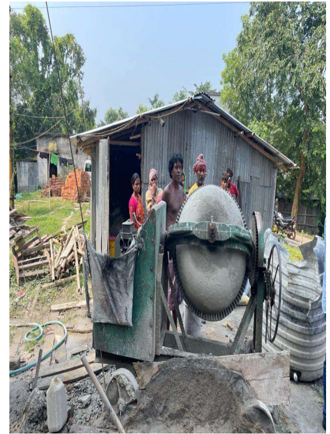
Ordinary concrete mixer in use
