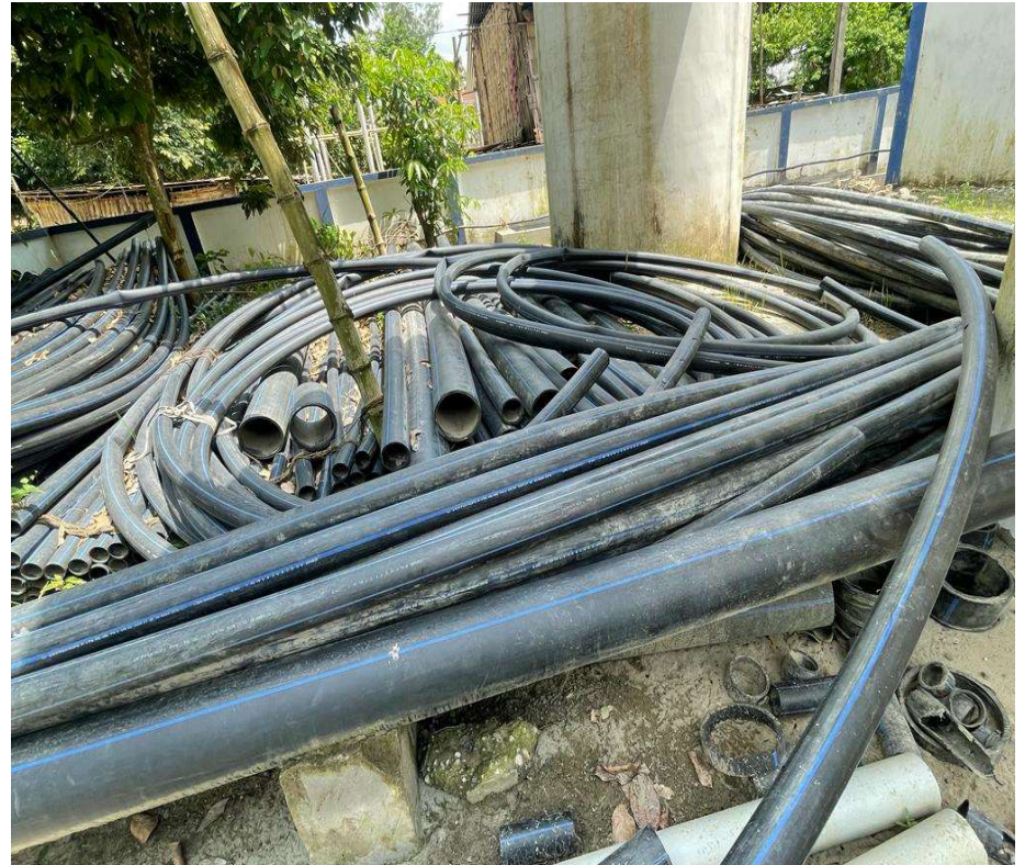
Improper stacking
