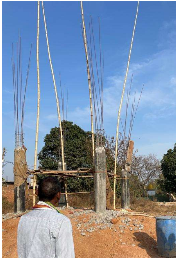
Poor concreting
