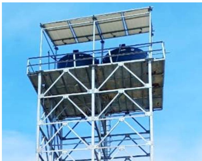
Figure 16: Solar pump-based water supply systems | Source: PHED, Chhattisgarh
