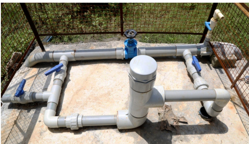
Figure 17: In-Line Chlorination device, set up by technical partner Evidence Action | Source: EA in Madhya Pradesh
