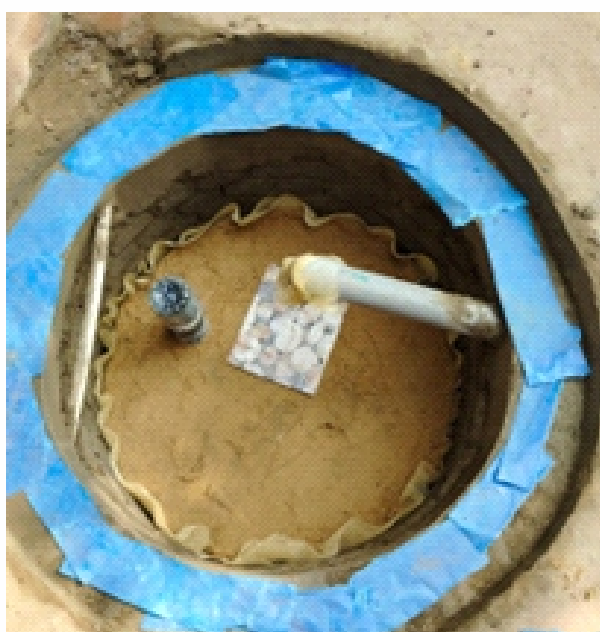
Replenishing groundwater through recharge shafts
