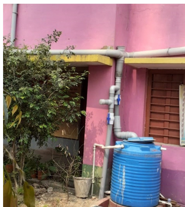
Rooftop rainwater harvesting system collecting precious water for use and groundwater recharge
