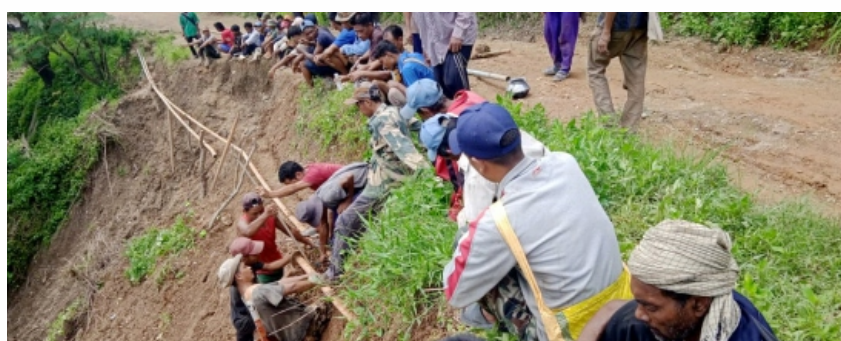
Hnatlang - Community participation realigning the gravity line damaged by a landslide, ensuring water supply restoration at Tuipubari village | Source: PHED Mamit
