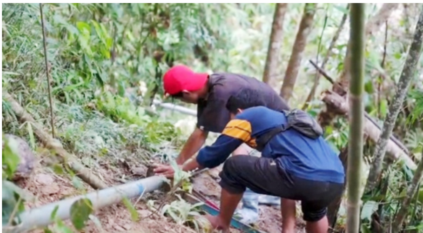
Figure 14: Laying of pipelines in hilly terrains Source: Basar PHE & WS Division, Arunachal Pradesh
