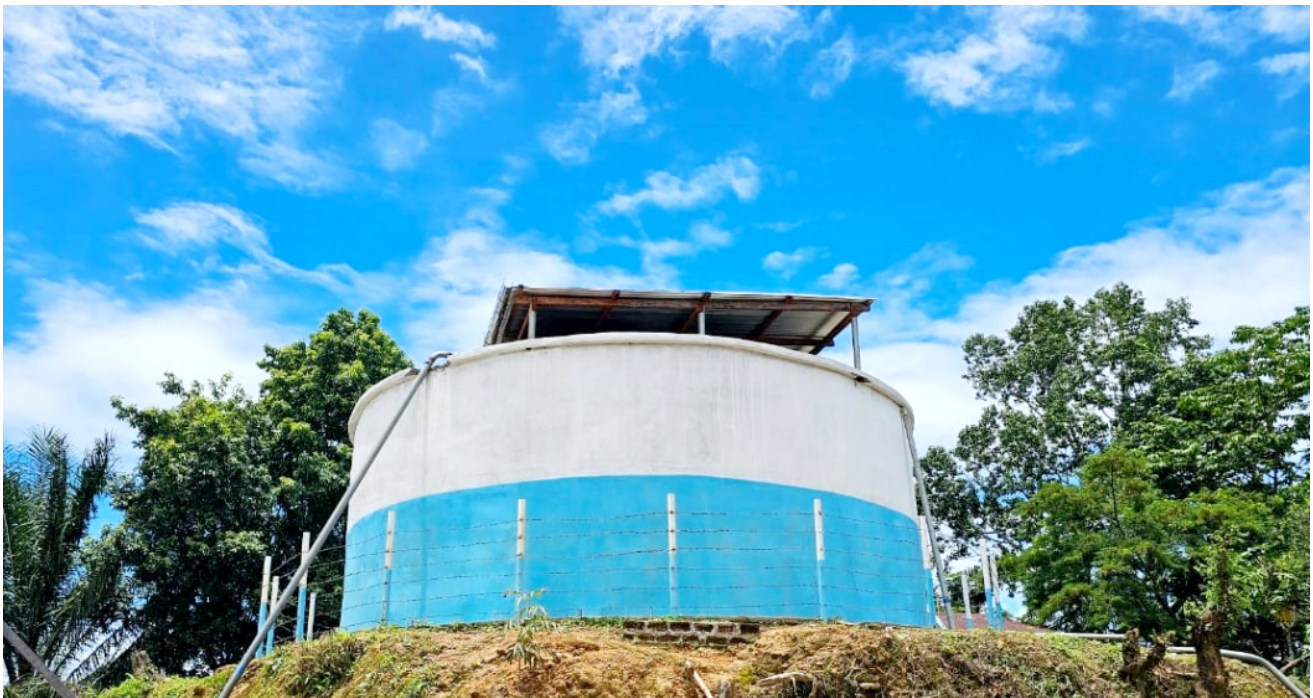
Figure 35: Rainwater Harvesting Structure on top of Existing Main Reservoir | Source: PHED Mizoram
