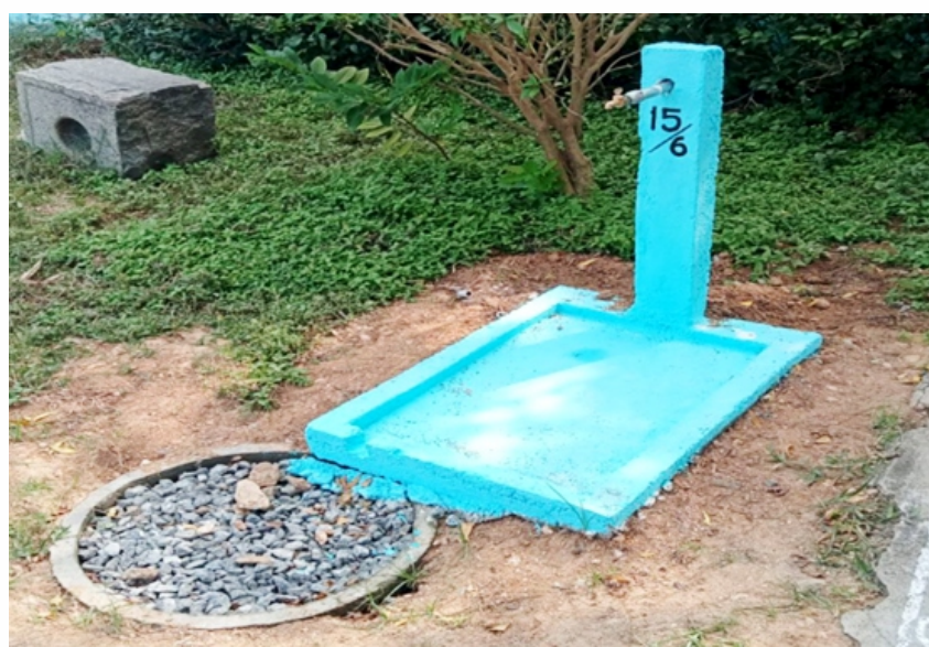
Figure 27: FHTC with soak pit | Source: RD Vellore
