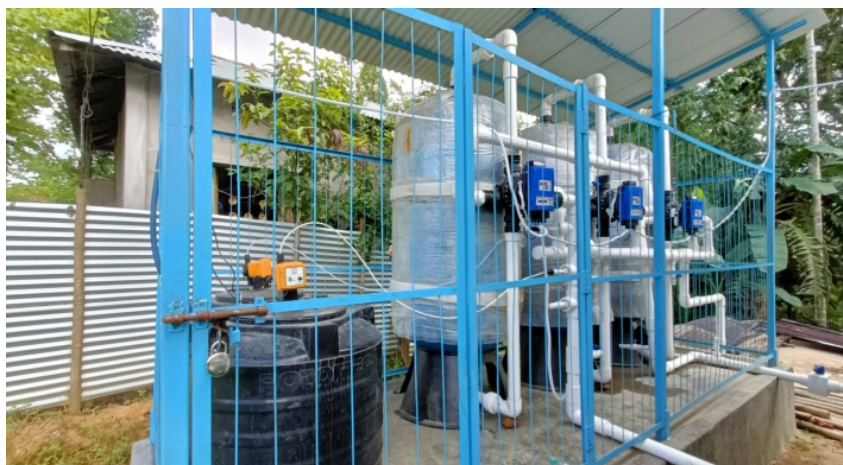
Figure 12: Halahali Iron Removal Plants (IRP) site | Source: CML
