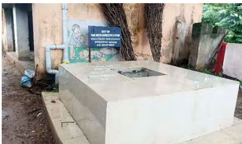
Figure 26: RTRWH Recharge Pit Langeswar High School Humma Burudi Ganjam | Source: UNICEF Odisha
