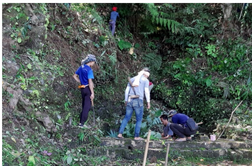
Figure 3-4: Cleaning of traditional water bodies to revive the sources | Source: PHED Nagaland
