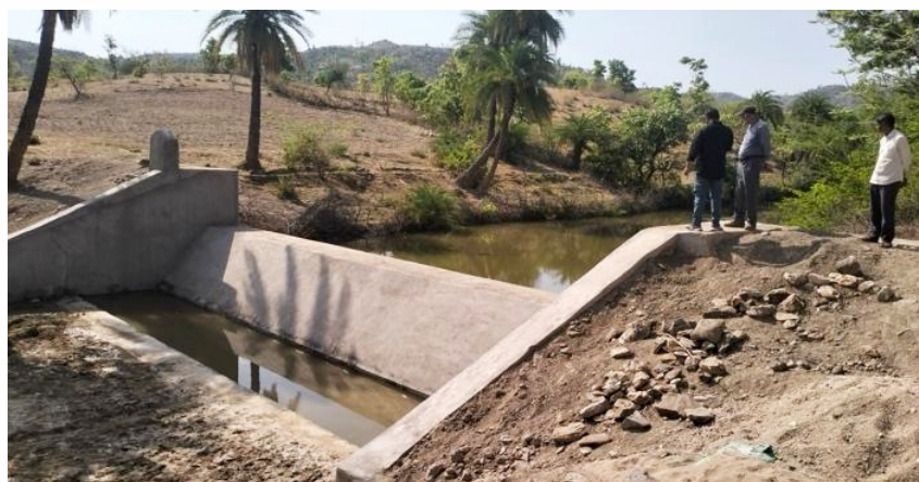
Figure 13: Check Dam Site | Source: CmF Tata Trusts
