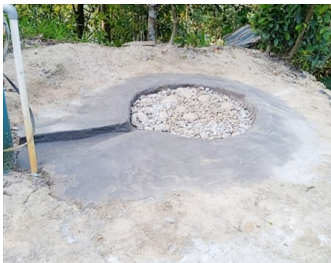
Figure 6-8: Recharge structures | Source: PHED Nagaland
