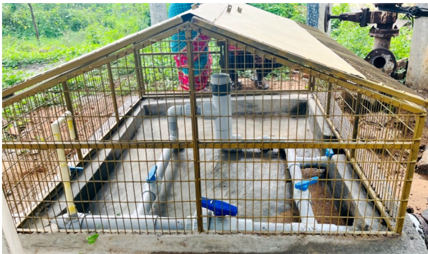
Figure 24: In-Line Chlorination (ILC) Device installed in the Thummalapalem Village, NTR District, Andhra Pradesh | Source: Andhra Pradesh EA team
