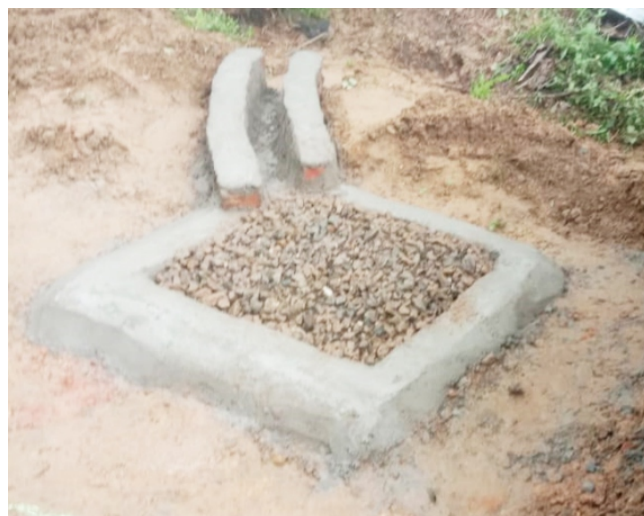
Figure 6-8: Recharge structures | Source: PHED Nagaland
