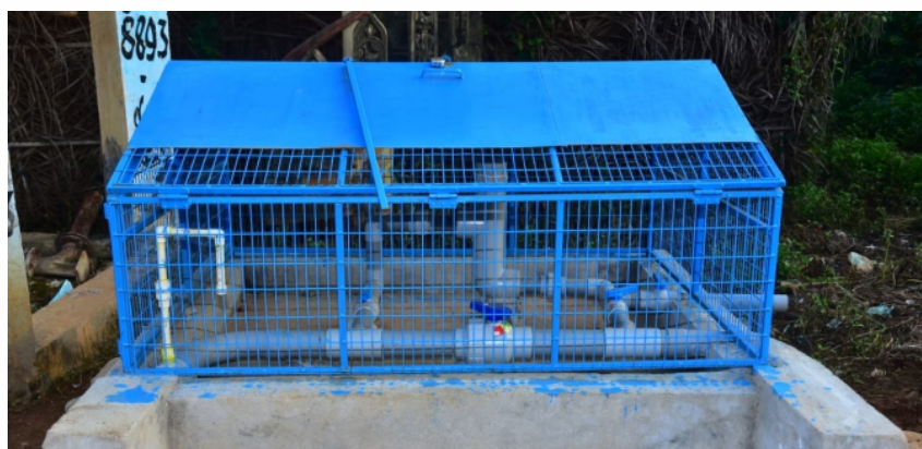
Figure 20: A In-Line Chlorination (ILC) device at Ramannagudem Village, Eluru District, Andhra Pradesh | Source: EA, AP
