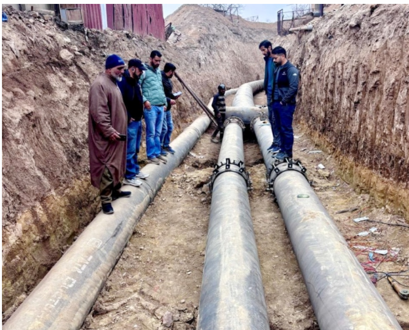
Figure 54: Hope glowing when Pipelines laying | Source: DWSM Baramulla
