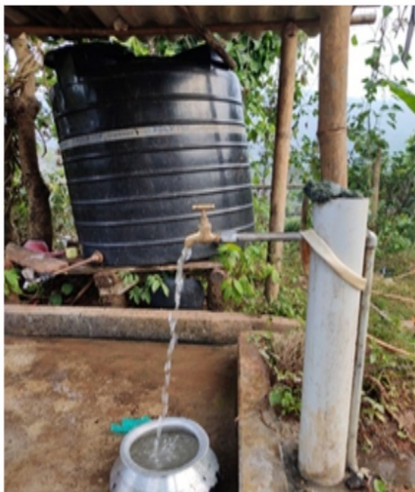
Figure 86: A functional household tap with storage tank | Source: DWSM Ri-Bhoi
