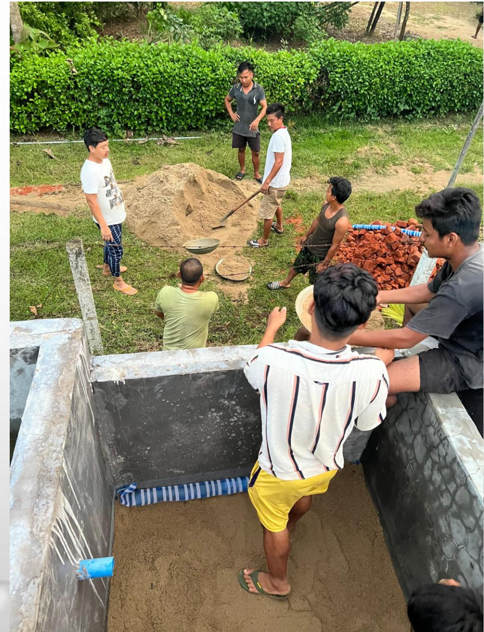
FILTER MEDIA FOR IRON REMOVAL PLANT BEING PLACED BY THE VILLAGERS
