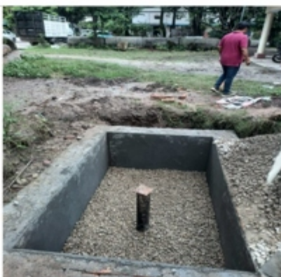
Figure 58-60: Water Harvesting structures | Source: DWSM Haridwar
