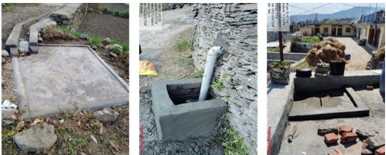
Figure 38-40: Community soak Pits covering end point discharge with community soak Pits (MNREGA+SBMG) | Source: DOWS, Tehri Garhwal
