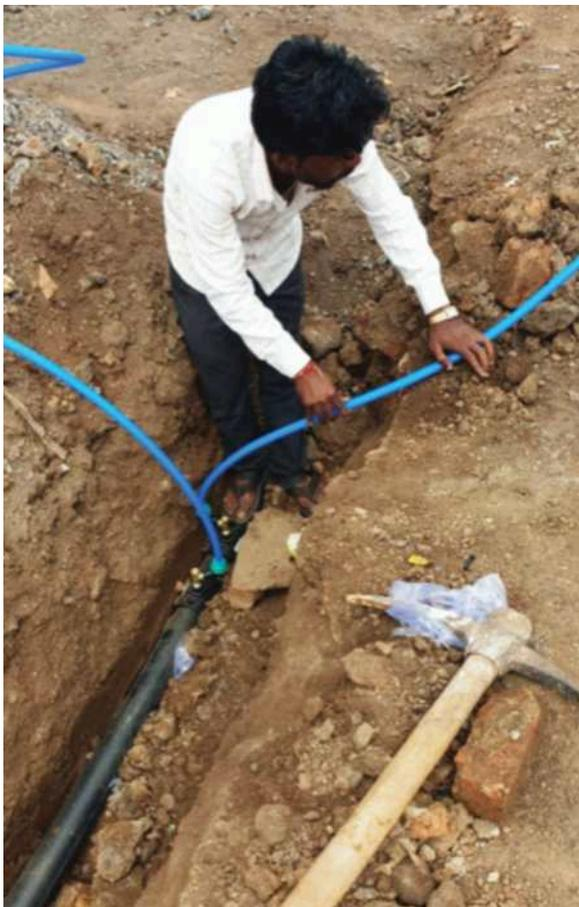
Providing saddle connection through electrofusion welding for household tap connection, Guna (M.P.)
