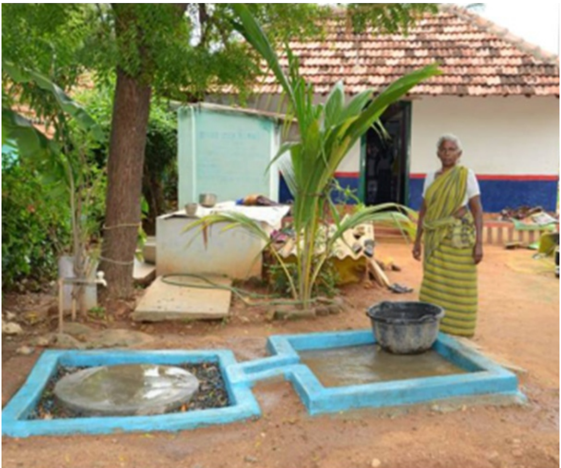
Figure 10: Soak pit for Greywater Management, Tamil Nadu
