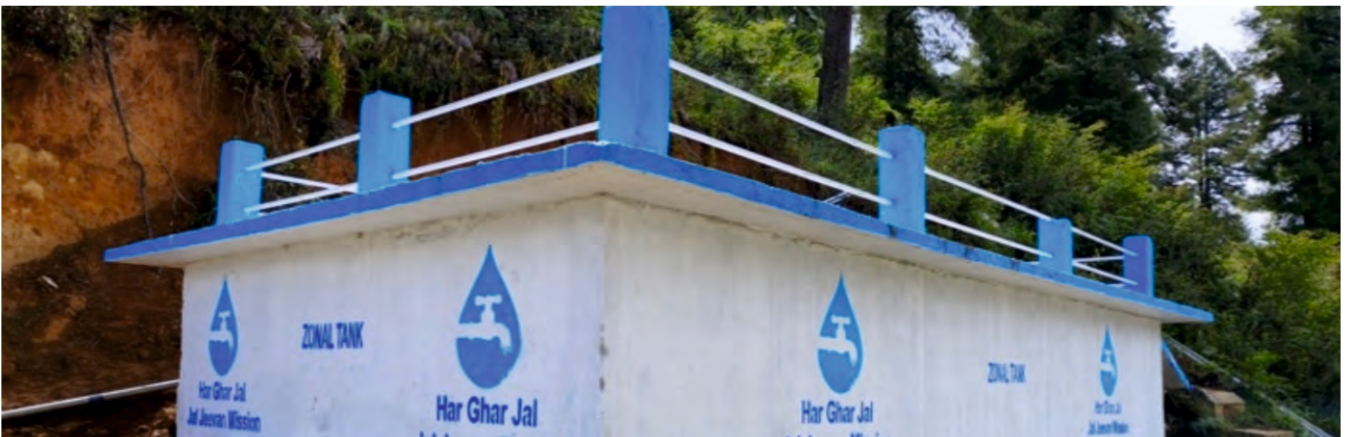
Pharge Village's Water Supply System under Jal Jeevan Mission Source: PHED, Arunachal Pradesh
