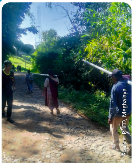
The community joins hands to carry pipelines
