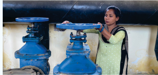
A VWSC woman member inspecting the main water line
