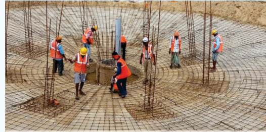
Rural youth being employed for infrastructure creation
