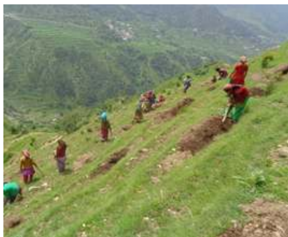
Photo 13: Recharge works through community participation in Tehri district of Uttarakhand
