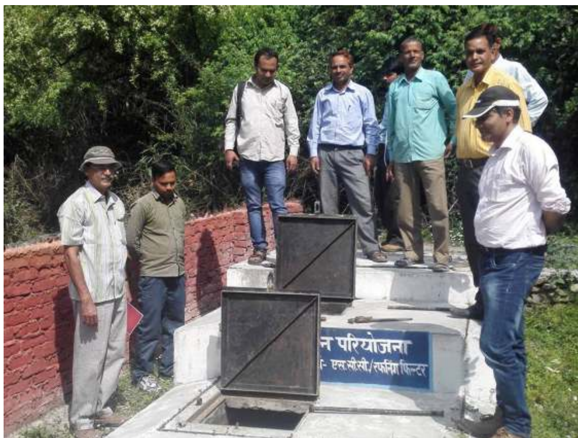
Photo 17 : Water collection chamber at Spring in Churedhar village of Tehri district of Uttarakhand
