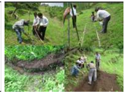
Photo 20: Recharge structure planning in the field
