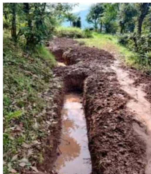
Photo 14: Groundwater recharge through contour trenches
