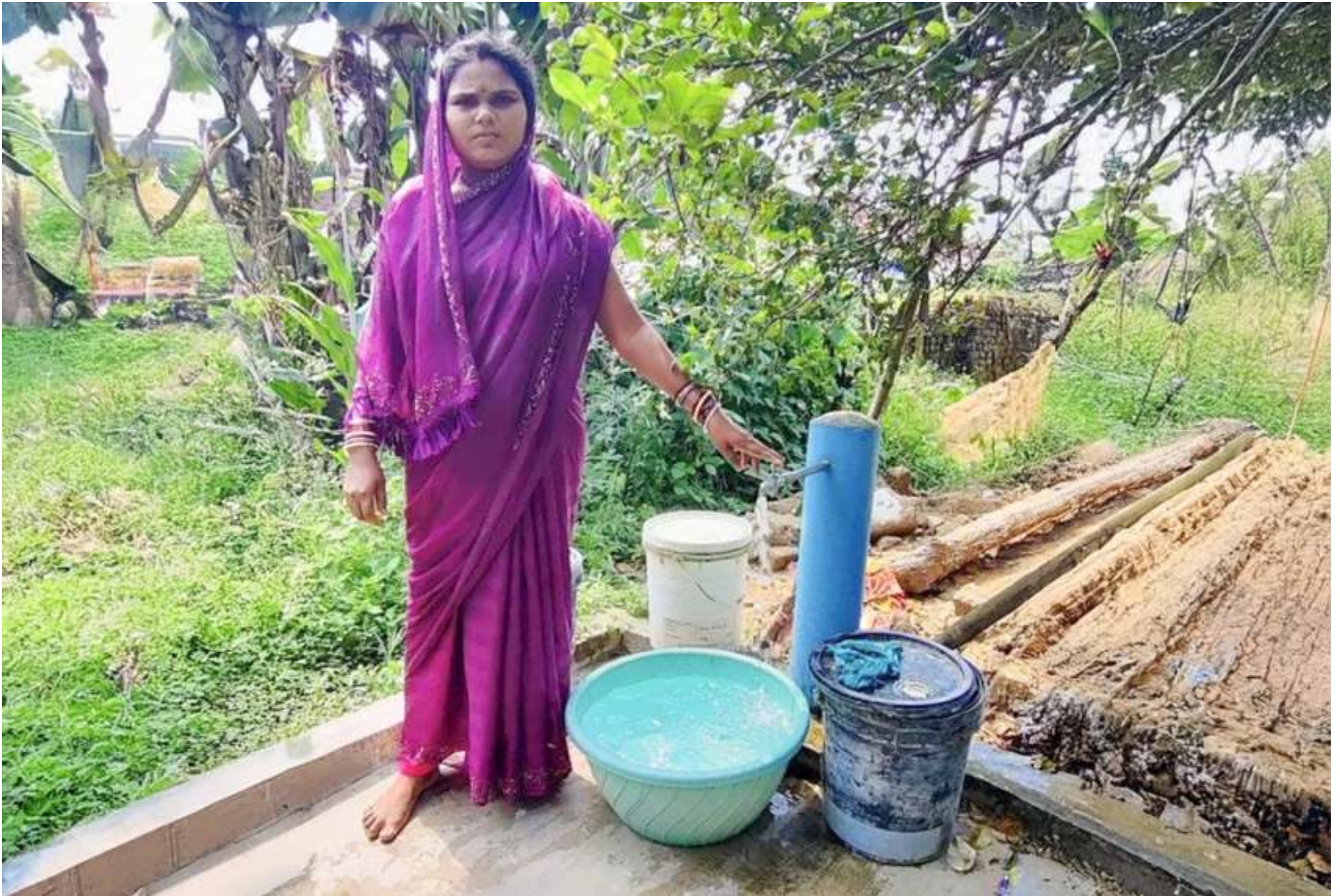
A woman proudly showcases a functional tap connection under JJM, ensuring clean and reliable water supply in her village | Source: PHED, Maharashtra
