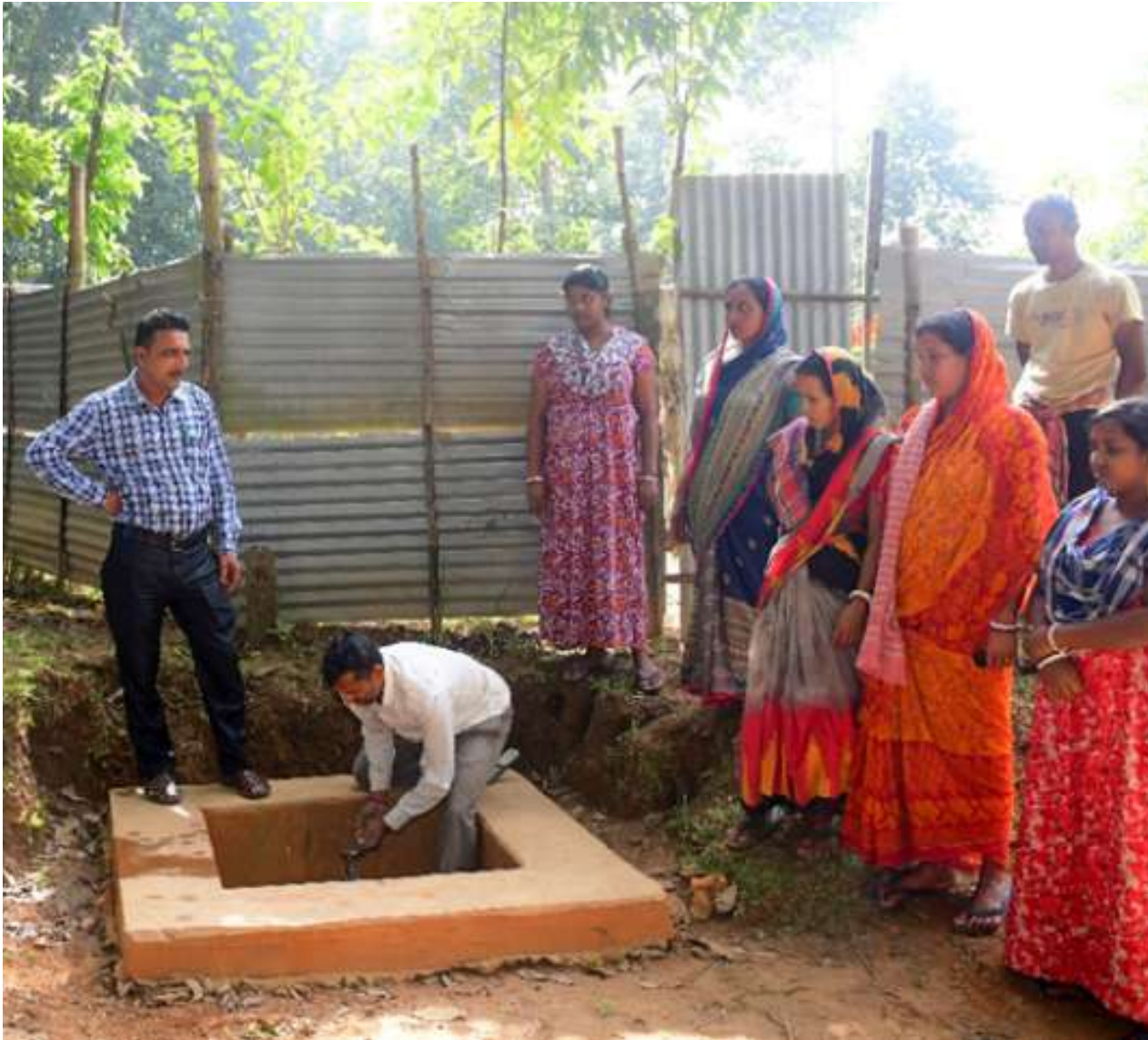
VWSC members monitoring work | Source: PHED Tripura
