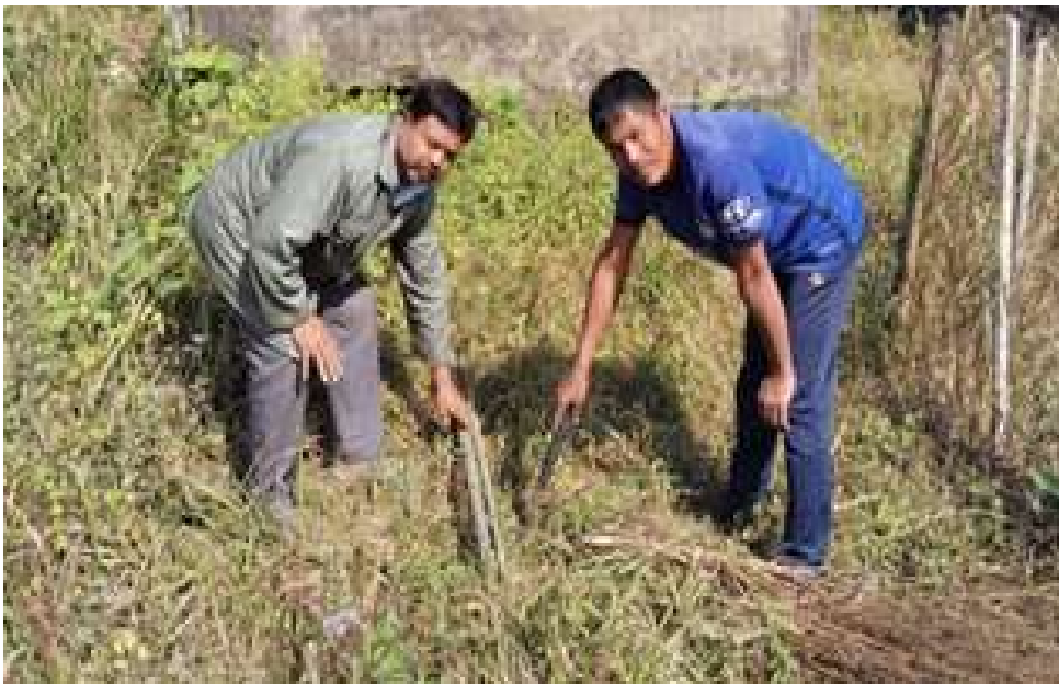
A beneficiary with Tap connection & Inspection of work | Source: PHED Meghalaya
