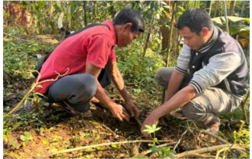
Images showing VWSC members repairing the pipes | Source: PHED Meghalaya
