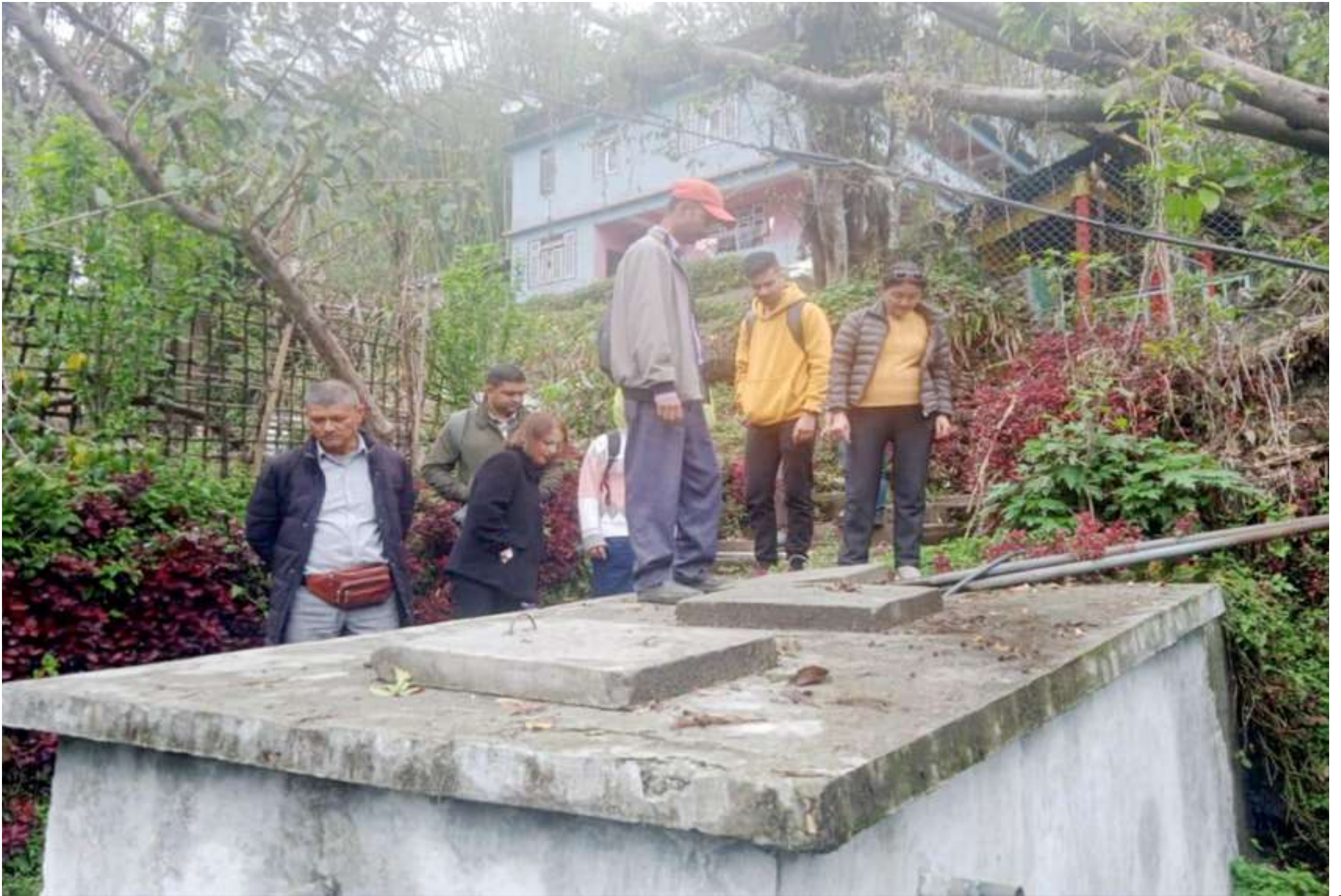
VWSC carrying out inspection of water tank | Source: RD, Sikkim
