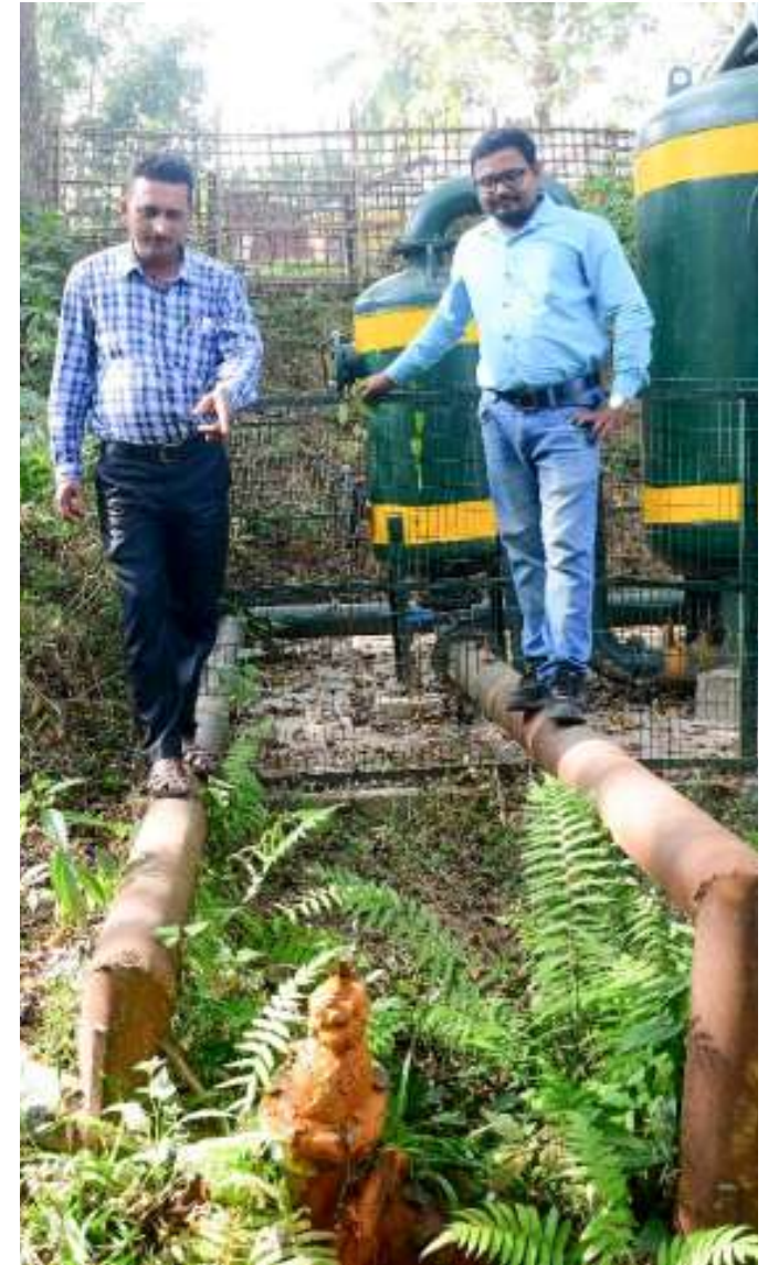
Inspection of water supply system | Source: PHED Tripura
