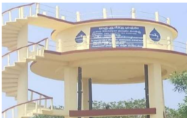
Overhead Storage Reservoir (OHSR) Source: RWS&S department, Andhra Pradesh
