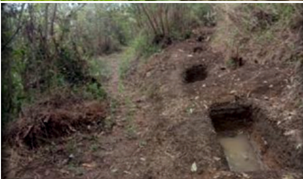
Contour trench constructed at the catchment area by the villagers.
