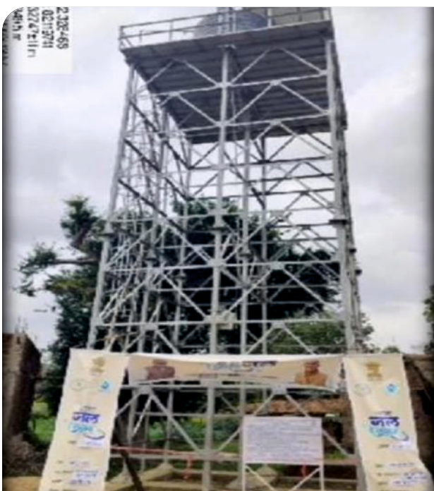
Solar based Overhead tank.
