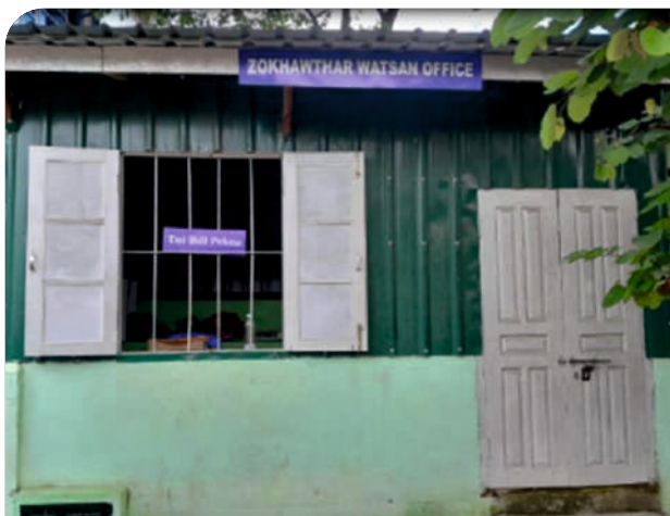
Zokhawthar's Watsan Office.
