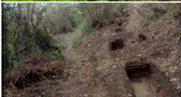
Contour trench constructed at the catchment area by the villagers.
