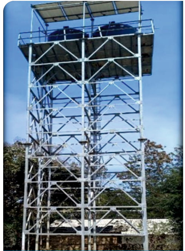
Solar pump-based water supply systems. Source: PHED, Chhattisgarh
