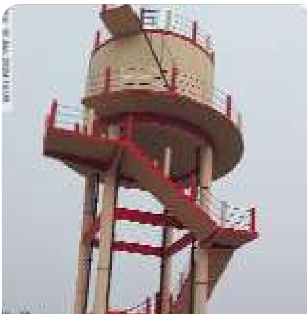
Construction of high level water reservoir Source: PHED, Chhattisgarh
