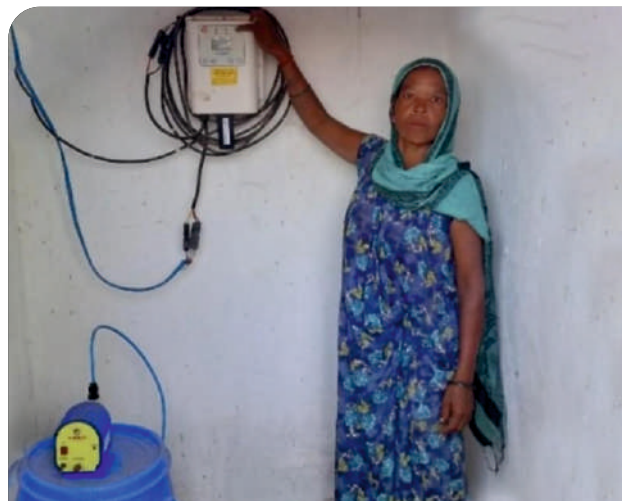
Storage tank constructed under the Jal Jeevan Mission
