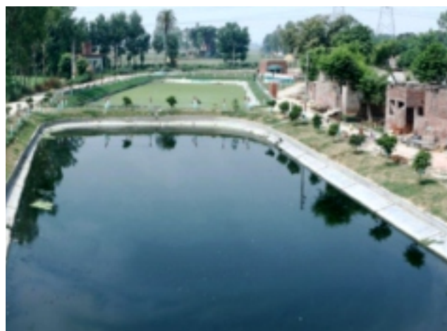
Waste stabilization pond in Karnal block, Haryana
