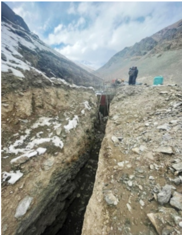
On going work in sub-zero temperatures of Ladakh
